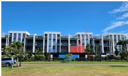
Unit 4, 10-14 Poinciana Blvd, Cardwell
